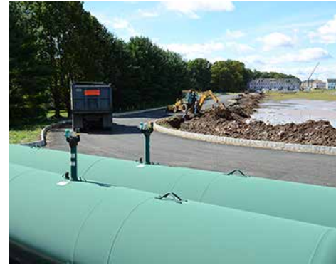
Carriage Hill's 563 condos, townhomes, and single-family houses are served by an individually metered central propane distribution system.
