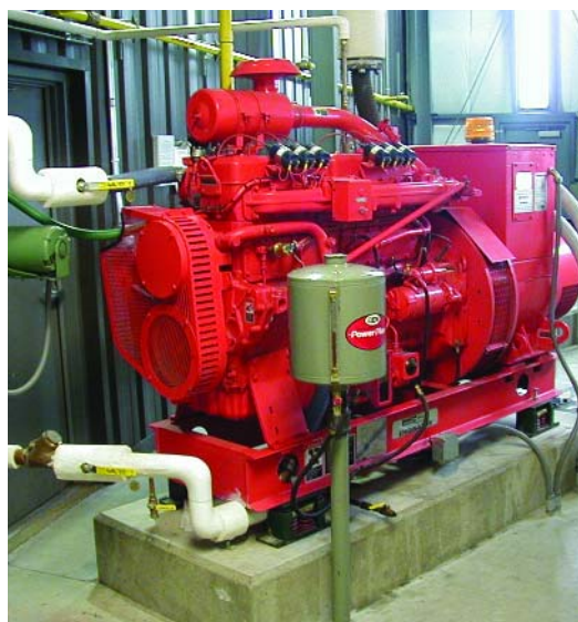
Northern custom designed this propane-fueled, combined heat and power system for Green Mountain Coffee Roasters.
